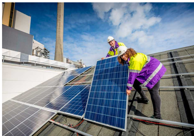
Figure 4. Installation of rooftop solar PV.
